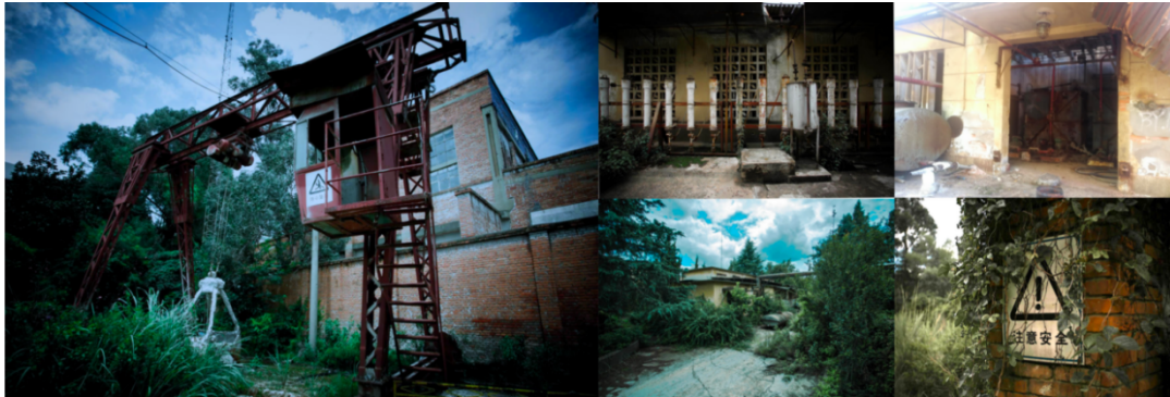
Image 1 Original spatial environment of Kunming Oxygen Plant (Source: Shicui Company)
