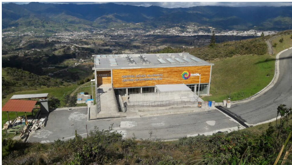
Figure A.13: Villonaco Wind Farm Visitor Centre.
