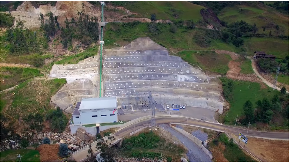
Figure A.17: Alazan hydroelectric power station site.
